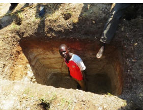
Digging the pit for the latrine.
