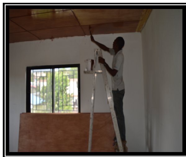
📍 Final touches on the ceiling
