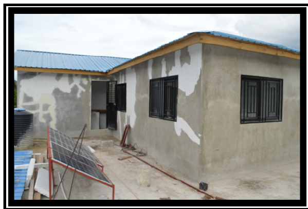
📍 Outside walls about to be painted
