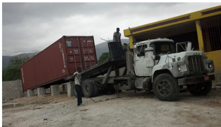
Grains storage silo made with a container
