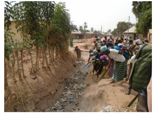
Beneficiaries work together to clean a drainage ditch filled with litter.
