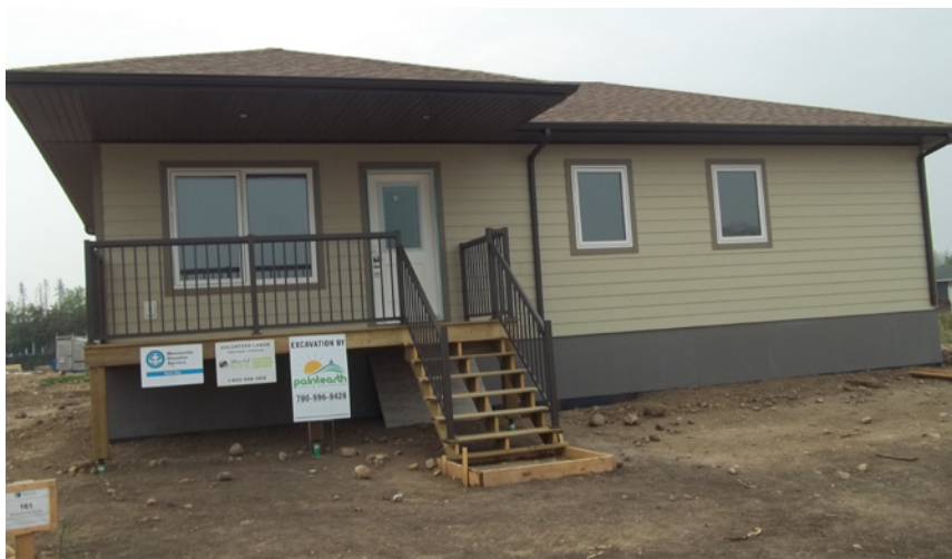
A home completed by volunteers from World Renew and Mennonite Disaster Services.
