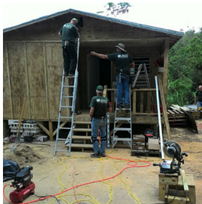
DRS volunteers work with local volunteers in Puerto Rico to build a house from the ground up.
