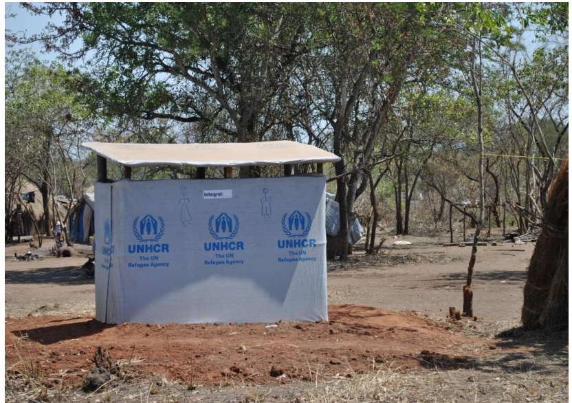
UNHCR tarps cover the latrines recently constructed by World Renew
