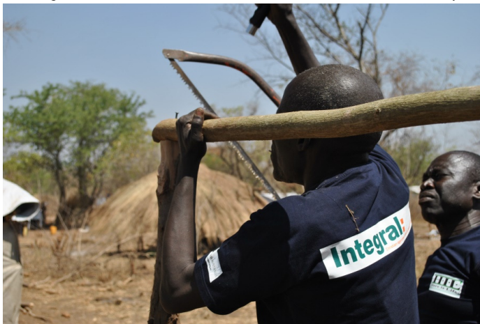
World Renew's local partner staff building latrines in Bidibidi refugee camp
