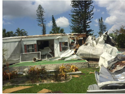
Home destroyed in Florida. FEMA News Photo
