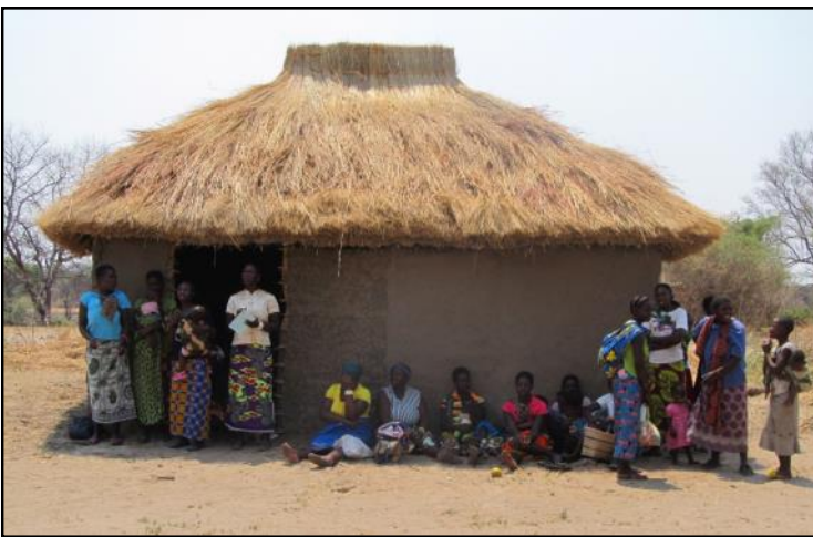
6. In Loanja, beneficiaries built a new storage building.
