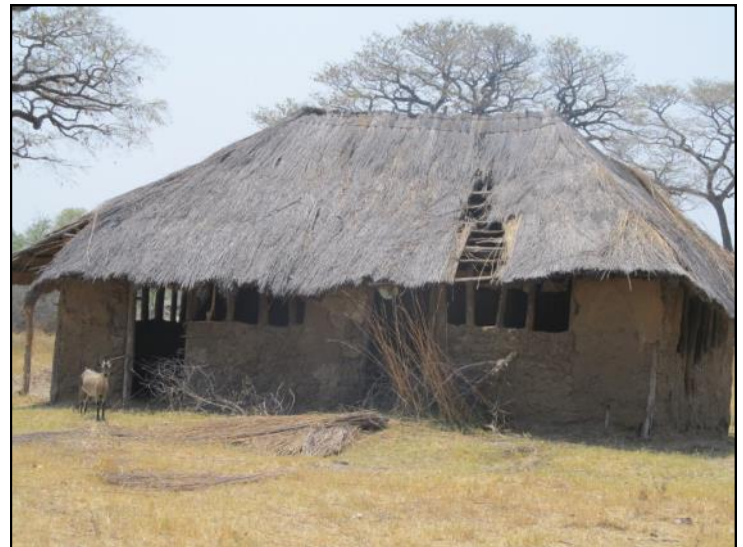
3. In Lutaba, beneficiaries will repair the roof on this building used for the school feeding program.
