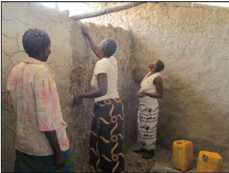
1. In Adonsi, beneficiaries mixed mud and applied it to the walls, to finish a home for two teachers.
