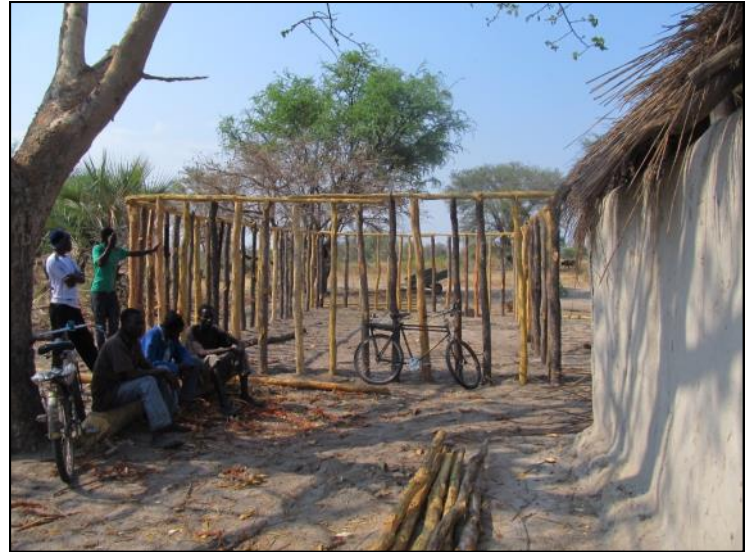
2. In Mabumbu, beneficiaries used traditional techniques to construct a building that can be used for storage of food when it rains and for community meetings.
